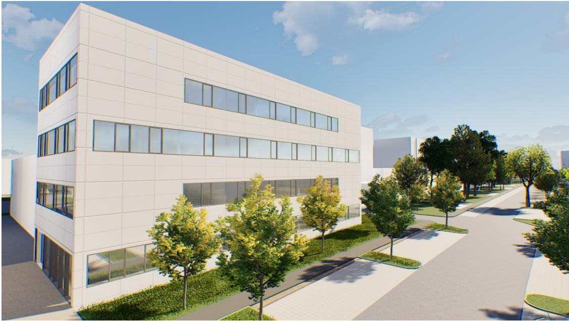
Image Source: Institute of Thermal Engineering, TU Graz
